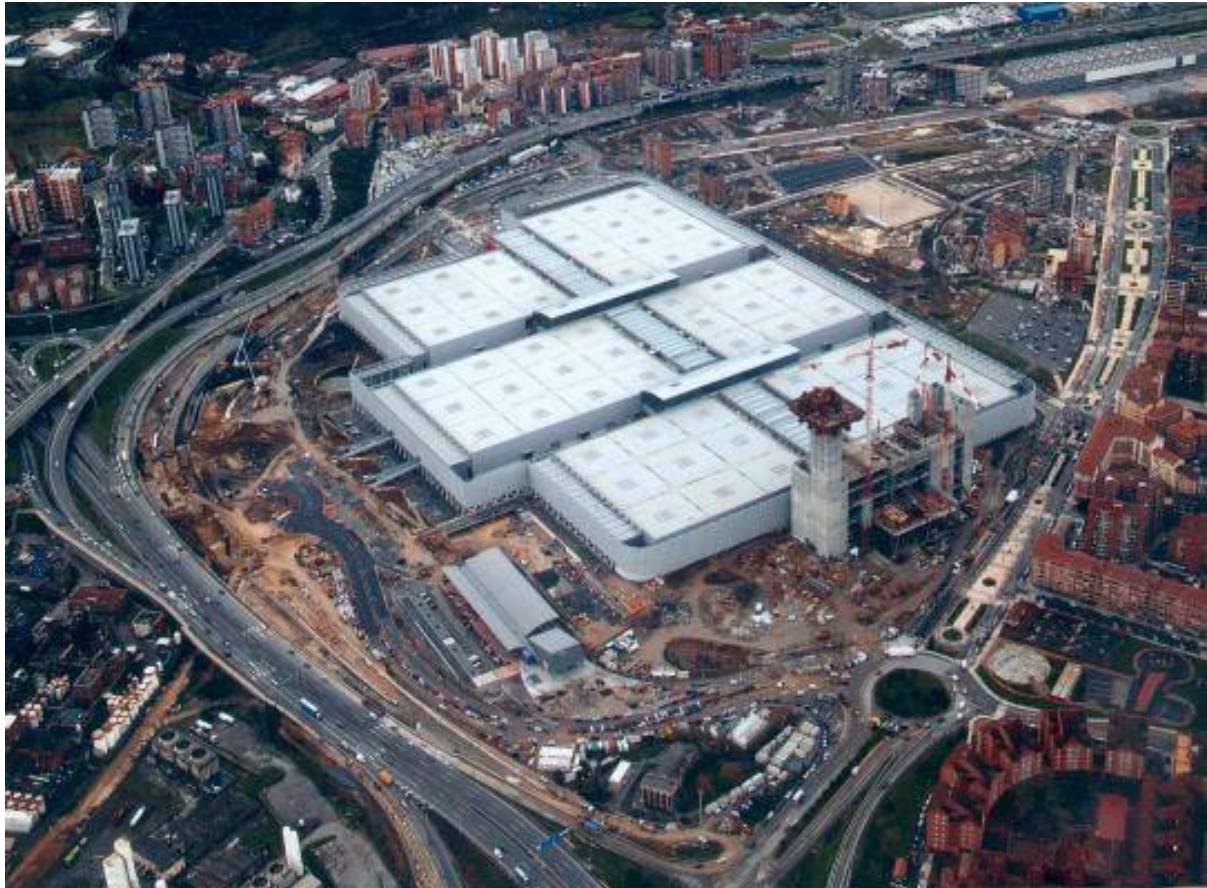
Bilbao Exhibition Centre - Vista aérea
